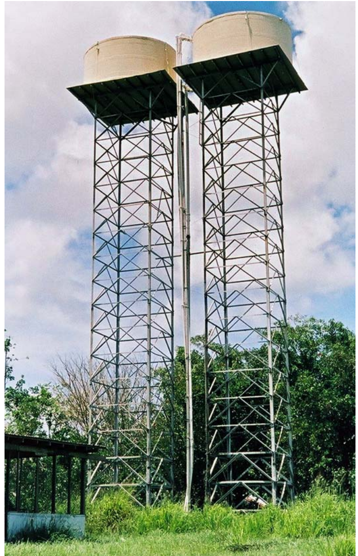
A water supply on Tonga: Rain and groundwater are stored in tanks and gravity fed to homes. (photo: Ilan Kelman).
