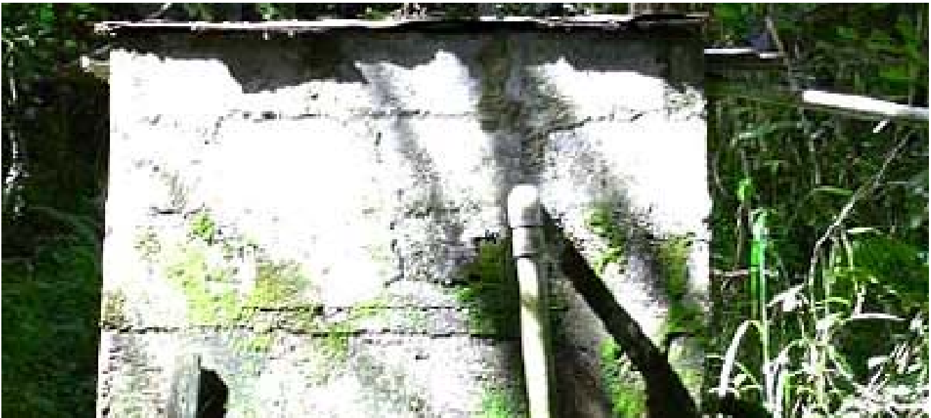
One drinking water system in a study site. The upper pipe takes stream water and gravity feeds it through the lower pipe to the houses below (photo: CECIA).
