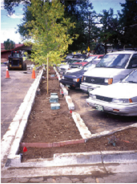
Stormwater runoff can be directed toward depressed, vegetated islands in parking lots, where trees can absorb and metabolize much of polluted runoff. The example here, at the corner of Baseline and Broadway, shows the construction process for such islands. Holes must exist in the curb for water to flow into, rather than around, the island.
