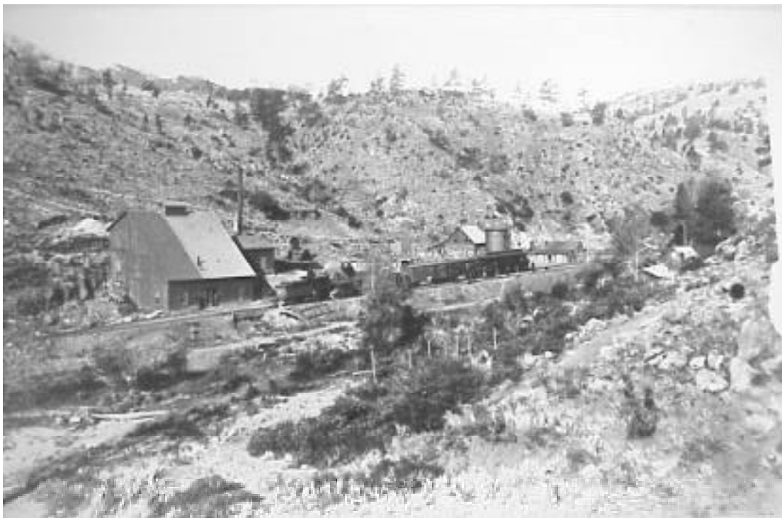
Town of Crisman, c. 1884 looking west toward Logan Mill. Notice how sparse the forest is on the hillside, compared with today. Before the miners settled in the district, natural ground fires kept the forest healthy. Miners cut trees for fuel, and by the time the forest grew back, our modern approach to fire suppression allowed much thicker growth. The result is an unhealthy thick forest that will burn fast and hot. Special thanks to Dee Bailey for providing the historic photographs.
